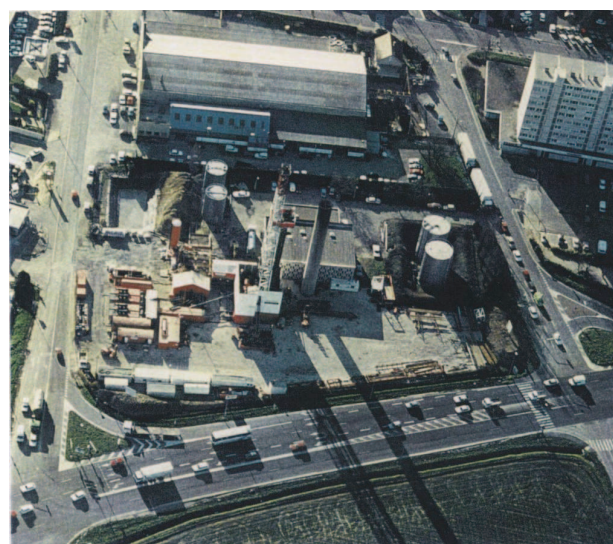
Fig. 4.2.3 – Geothermal drilling. Melun. France (source: GPC/Sedco-Forex)
